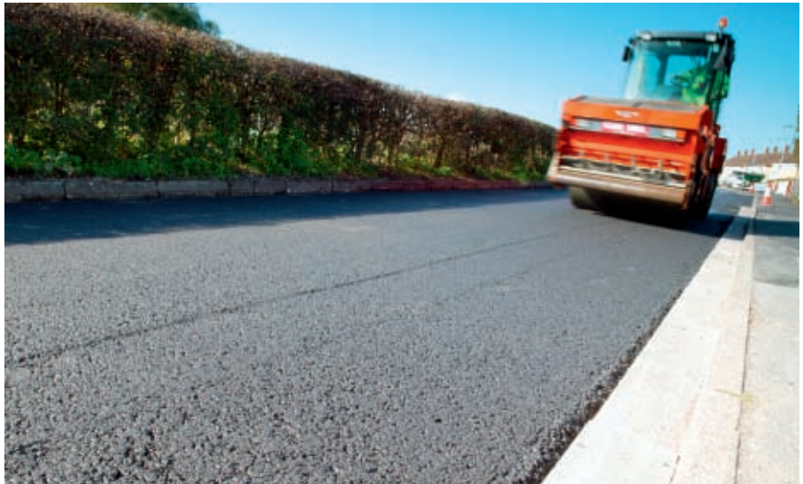
Materials produced to the Low Energy Asphalt process are like for like replacements for standard base and binder courses. The technology has not yet been applied to surface course mixes in the UK
